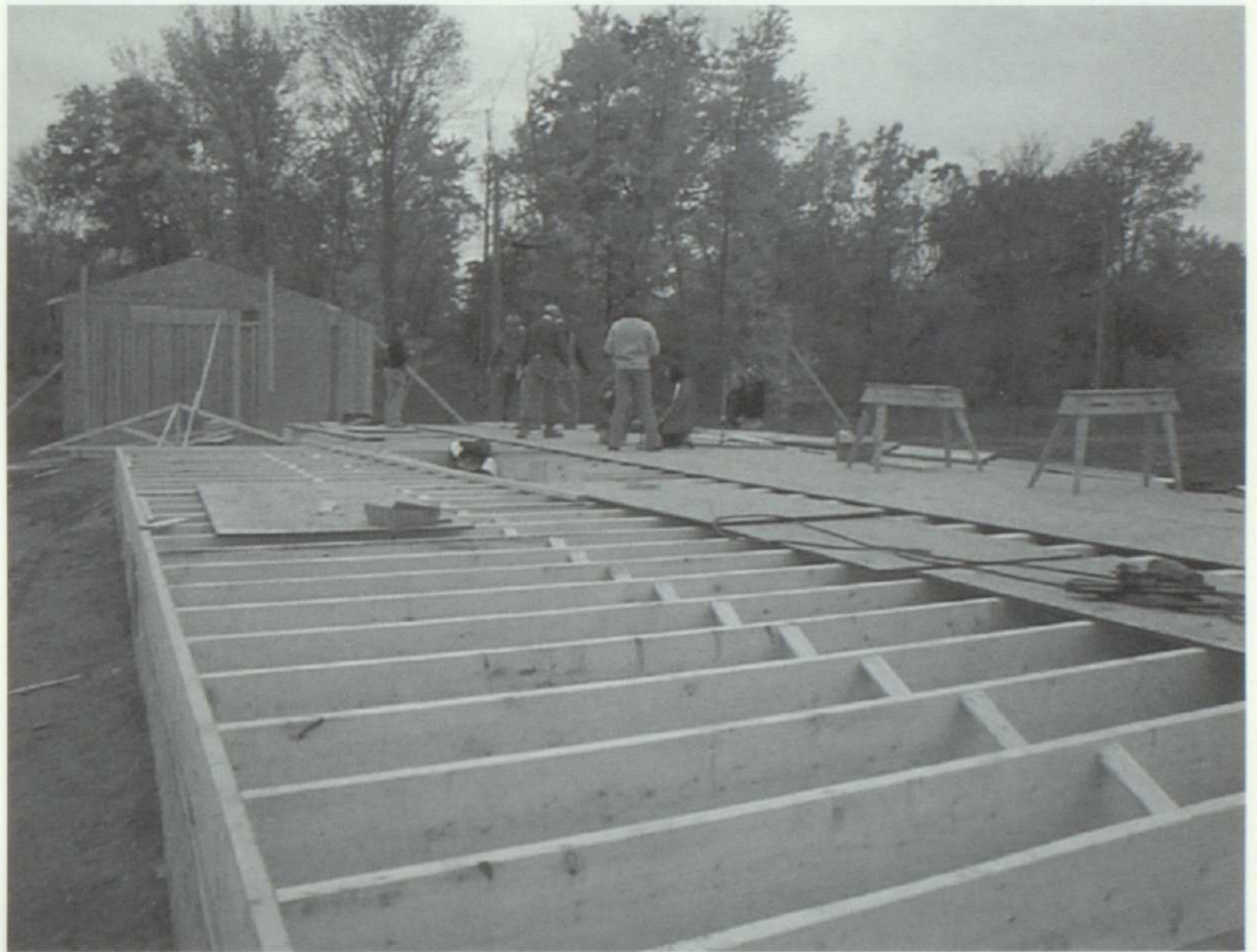
The class is just beginning the floor framing of the Home B.A.S.E. home. It is not as easy as it appears!
